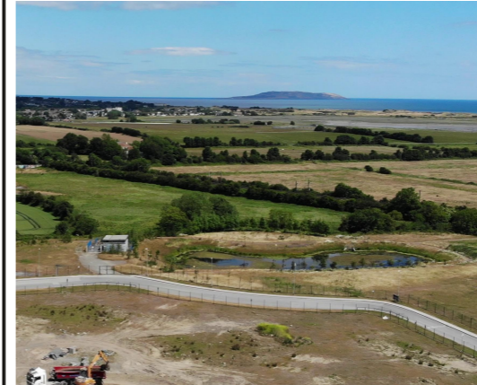
Attenuation pond and Wetland Park under construction
