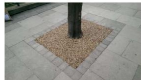
Resin Bond Tree Pit'
