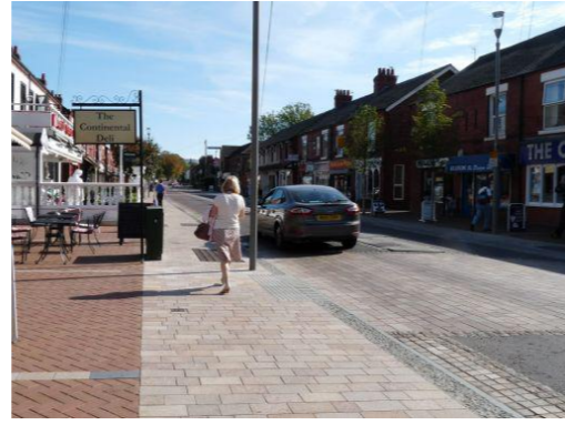
Flush surfaces encourage driver caution
